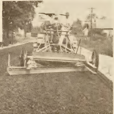
BELOW: THE DRAG PROVED VERY SATISFACTORY FOR SMOOTHING THE SURFACE AFTER THE MIXING OPERATION WAS COMPLETED
